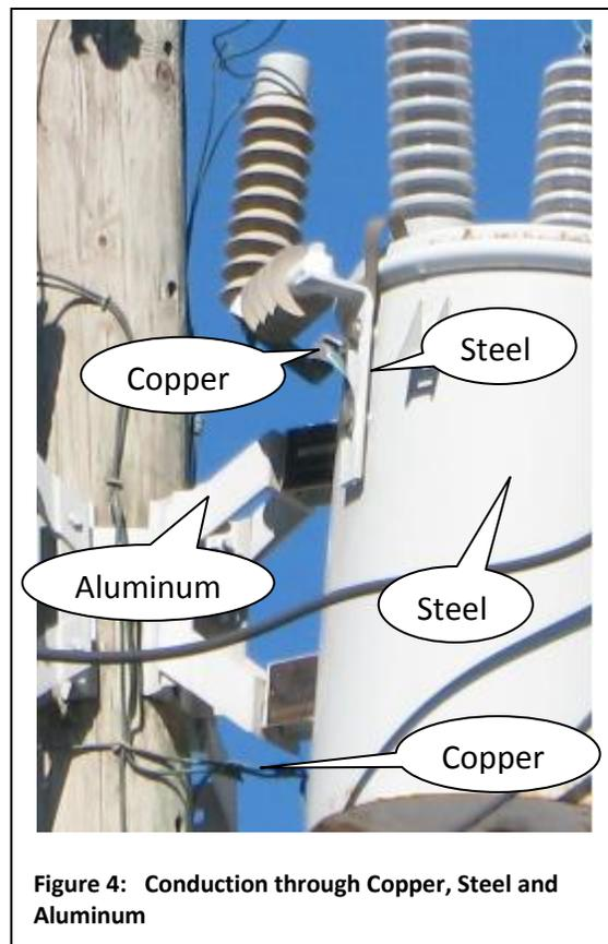
Figure 4: Conduction through Copper, Steel and Aluminum
