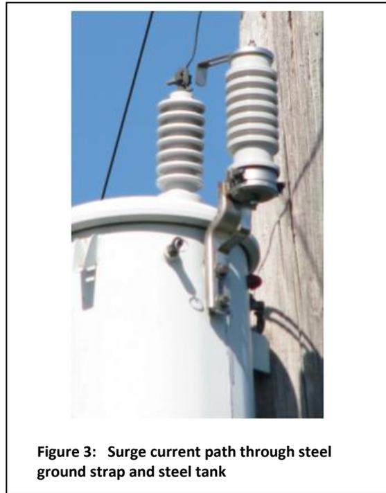
Figure 3: Surge current path through steel ground strap and steel tank
